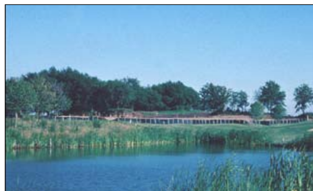
Naturalized detention area (Mill Creek Subdivision, Geneva, Illinois).
