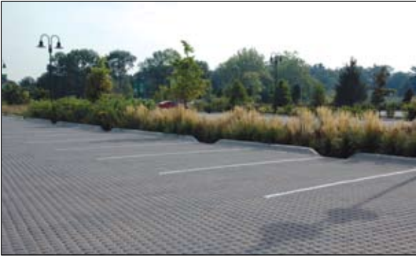
Porous Pavement Example 2: Another type of porous pavement features pavers to allow for immediate infiltration (Morton Arboretum, Lisle, Illinois).
