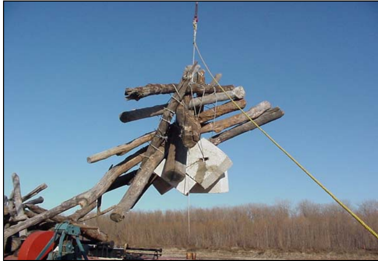
Photograph 4-9. Timber Piles Used to Provide Structural Depth Diversity and Island Protection
