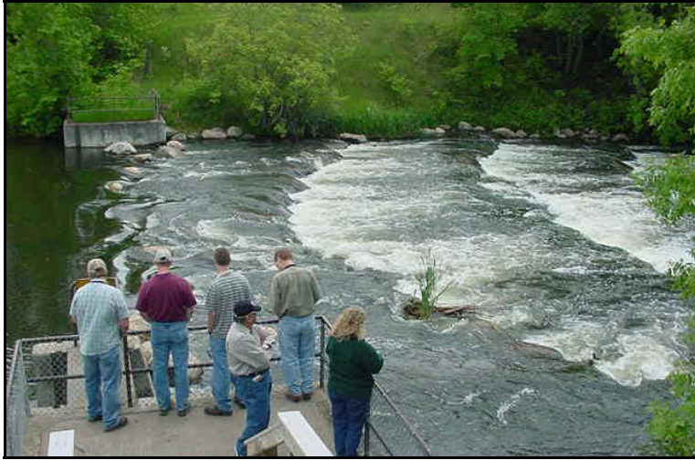
Photograph 3-5. Rock Ramp- Otter Tail River, Minnesota
