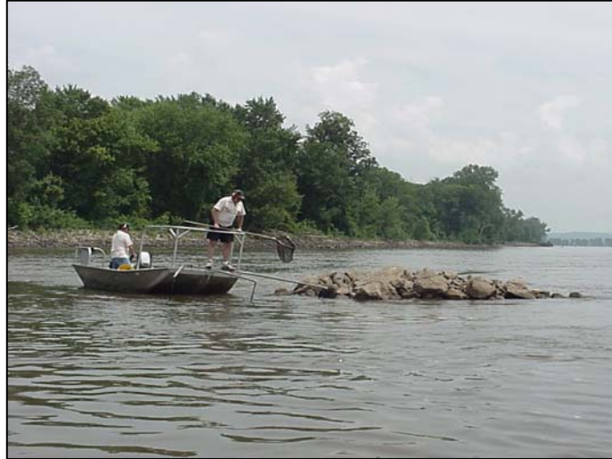
Photograph ES-2. Example of Instream Rock Pile Structure
