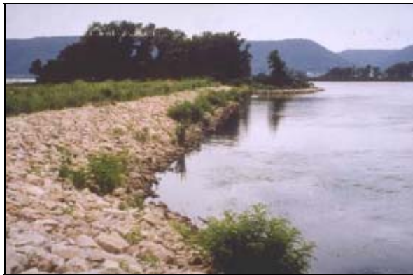
Photograph 4-2. Rock Revetment Used for Bank Stabilization
