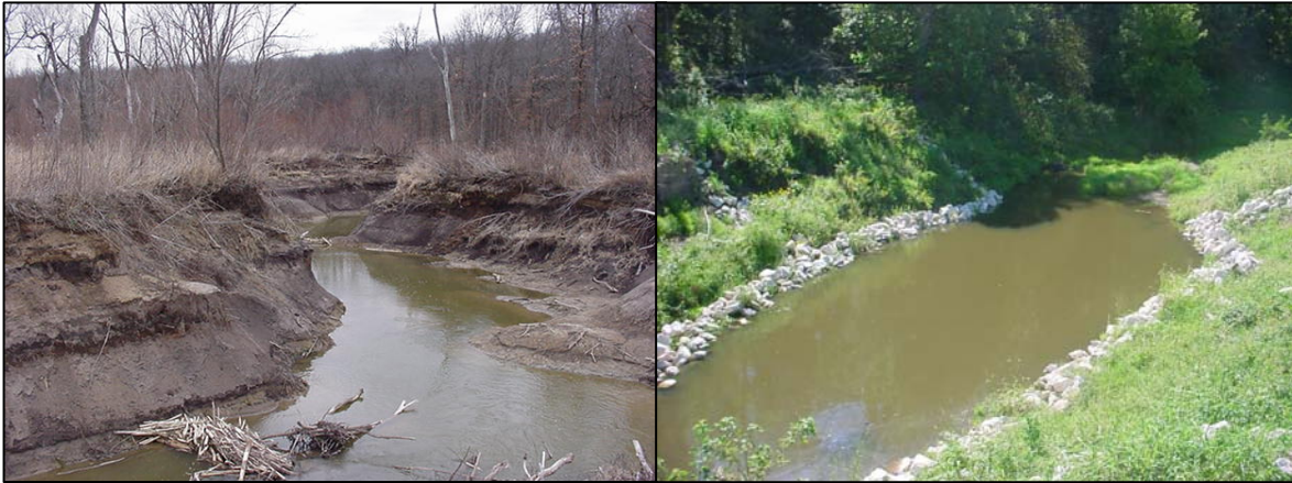
Photograph ES-1. Example Before and After Stream Restoration With Stone Toe Protection
