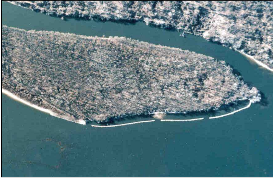
Photograph 4-10. Off-Bank Revetments Used To Provide Erosion Protection on Islands
