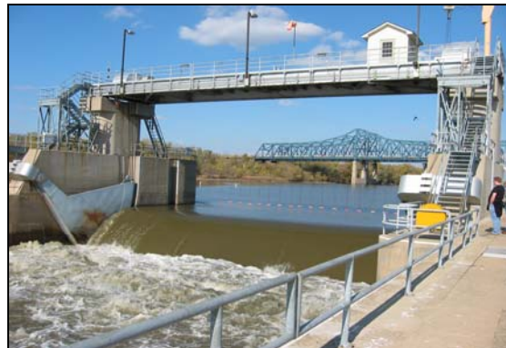
Photograph 3-9. Existing Tainter Gate at Peoria Lock and Dam
