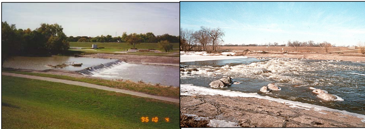
Photograph ES-4. Before and After Rock Ramp Fish Passage at a Low Head Dam
