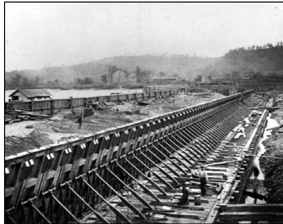
Photograph 3-8. Construction of Wicket Dam on the Ohio River
