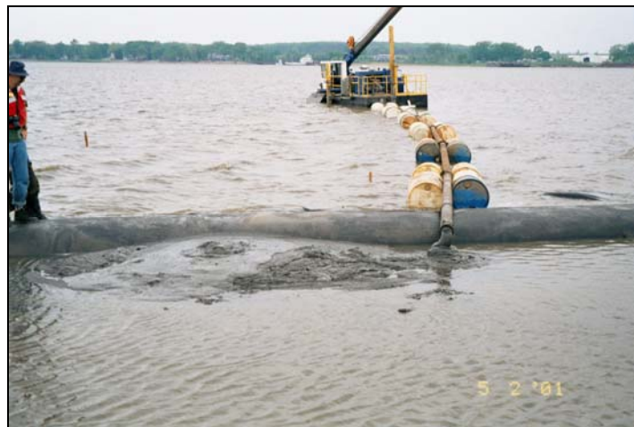
Photograph 4-7. High-Solids Dredging Technology Used Where Fine-grained Sediments Are Prevalent
