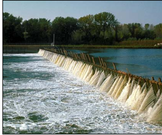
Photograph 3-7. Existing Wicket Dam at Peoria Lock and Dam
