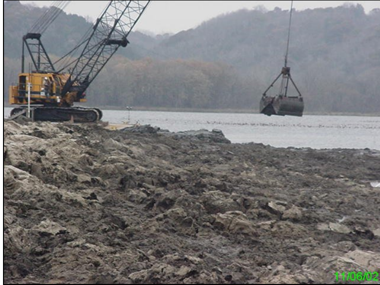
Photograph 4-6. Island Creation Utilizing a Clamshell Bucket To Mechanically Dredge Sediment
