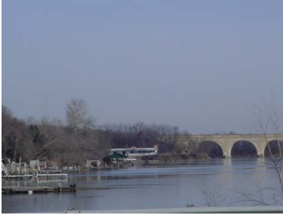
Lake Decatur at Williams Street Looking North
