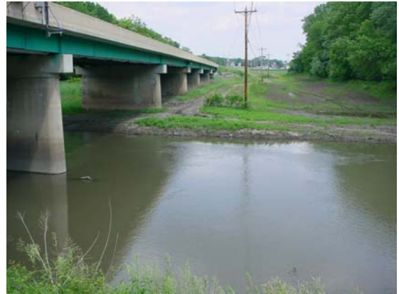
Sangamon River Segment E29 at Route 136 Looking East
