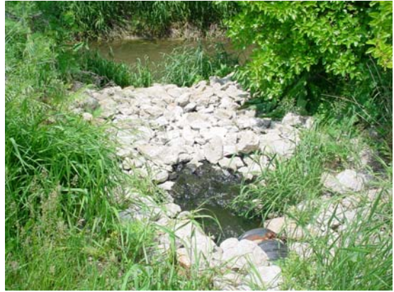
Fisher Sanitary Treatment Plant Discharge (to Owl Creek)
