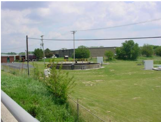
Fisher Sanitary Treatment Plant
